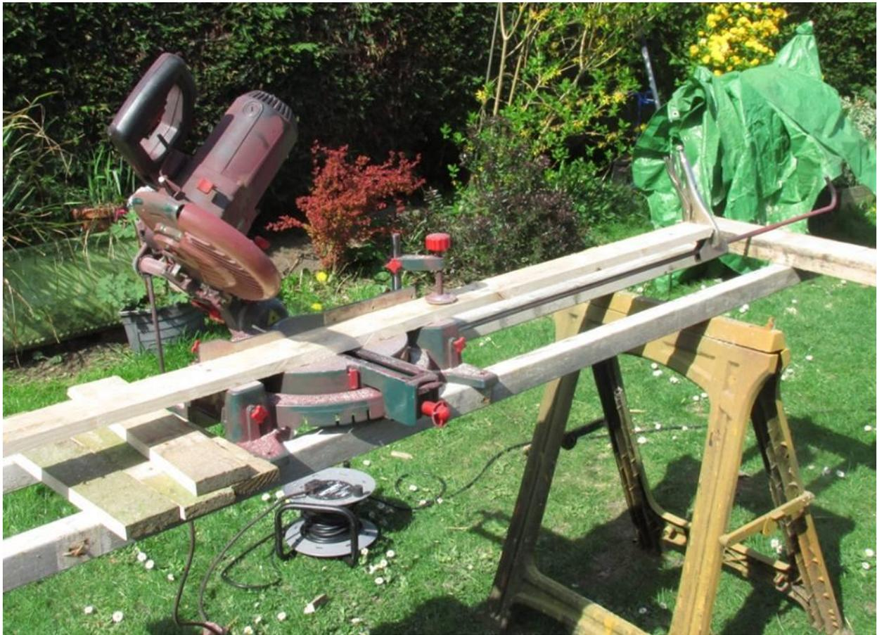
30 boards which is sufficient to make 3 GrowBag boxes all cut to length with mitered ends and stacked up ready for receiving a couple of coats of raw Linseed oil.
