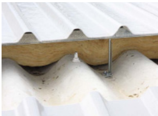
Picture 2 Bar & bracket with sheet and insulation
