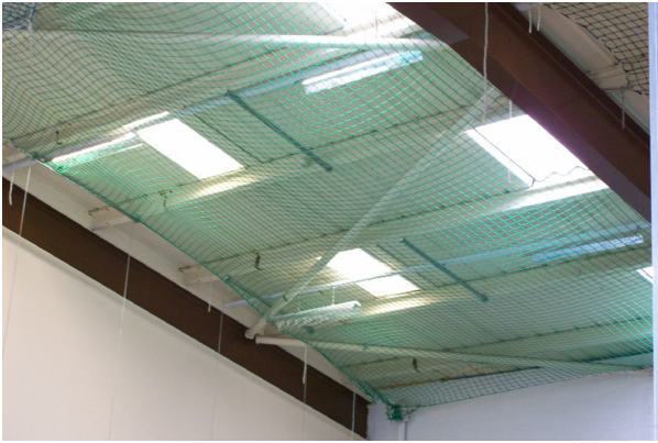
Picture 5 Close hung internal safety nets
